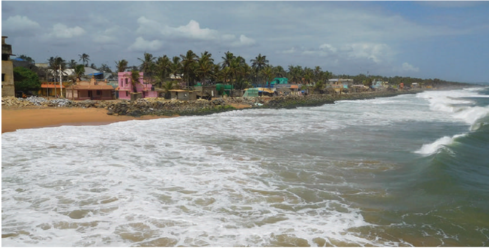
Fig 7.1: A view of the Valiyathura village from the top of the pier. Photo credit: TA Ameerudheen
