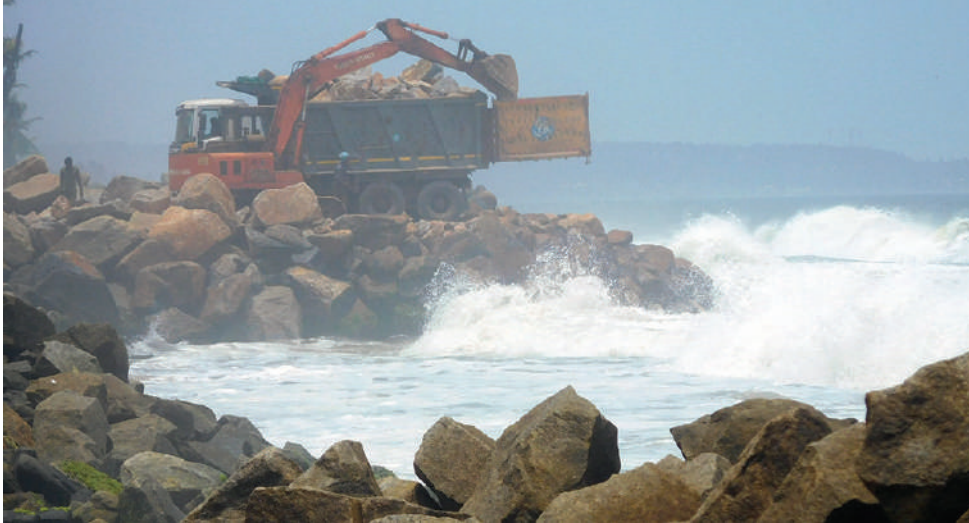
Groyne construction in progress in Valiyathura.
