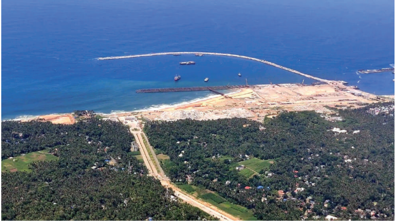
Aerial Photo of Vizhinjam International Seaport taken 21 September 2023
