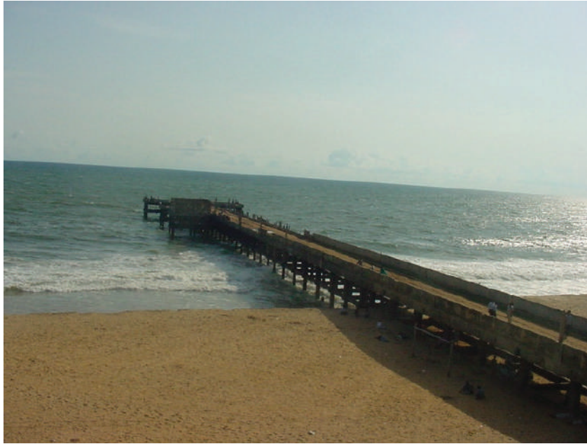
Fig. 5.15. Wide beach and the pier at Valiyathura prior to commencement of port construction
