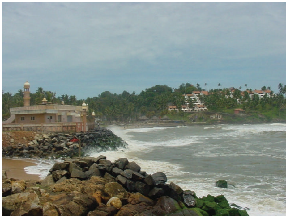
Fig. 5.7. Kovalam - Once there was a very wide beach seaward of the building (even during monsoon season) which was built (in 1984) landward of the monsoonal berm crest – best example of what happens with interventions on beach processes (Credit: K V Thomas)
