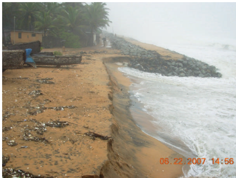
Fig. 5.9a. Low seawall with beach on its seaward side even during monsoon at Valiyathura (Photo: June 2007)
