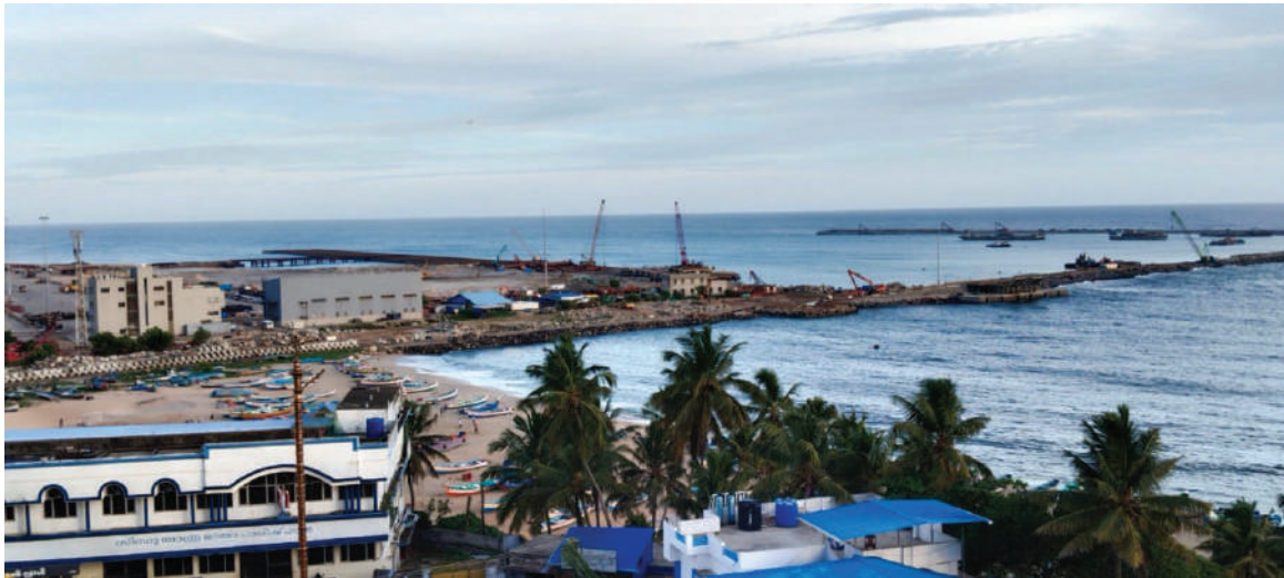
Fig 11.1: VIS Breakwater as on June 3, 2023
