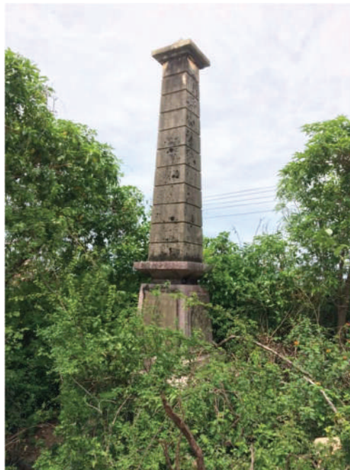
Fig 2.4: Pillar elected when starting the Vizhinjam Fishing Harbour construction Credit: Alphonsa Joseph
