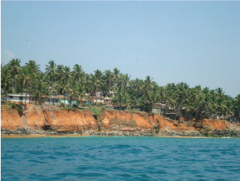
Fig 3.2: Eroding cliffs (photo of 2013) south of Vizhinjam Fishing harbour and very close to VIS site and toe protected by seawalls – Still the EIA claimed Vizhinjam and adjoining coasts as stable (Credit: Cyriac Kodoth)
